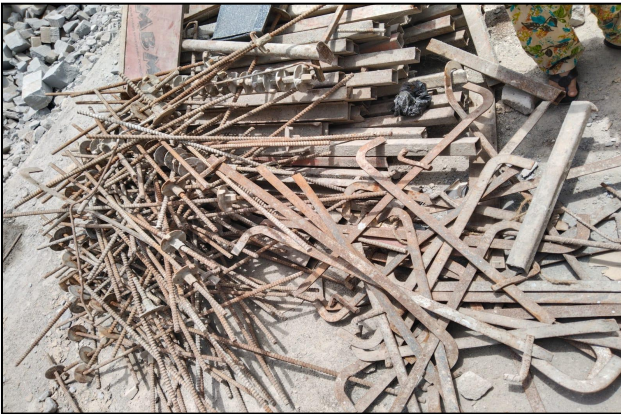
Steel used in Formwork
