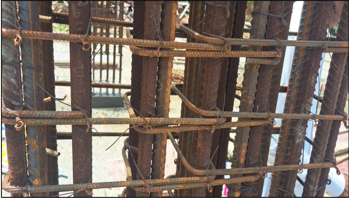
Binding of Steel using Bent up Bars
