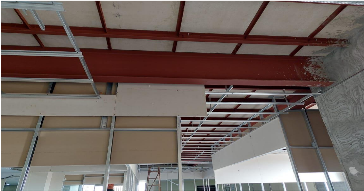
Different Steel cross sections ( I , Channel, Angle)
