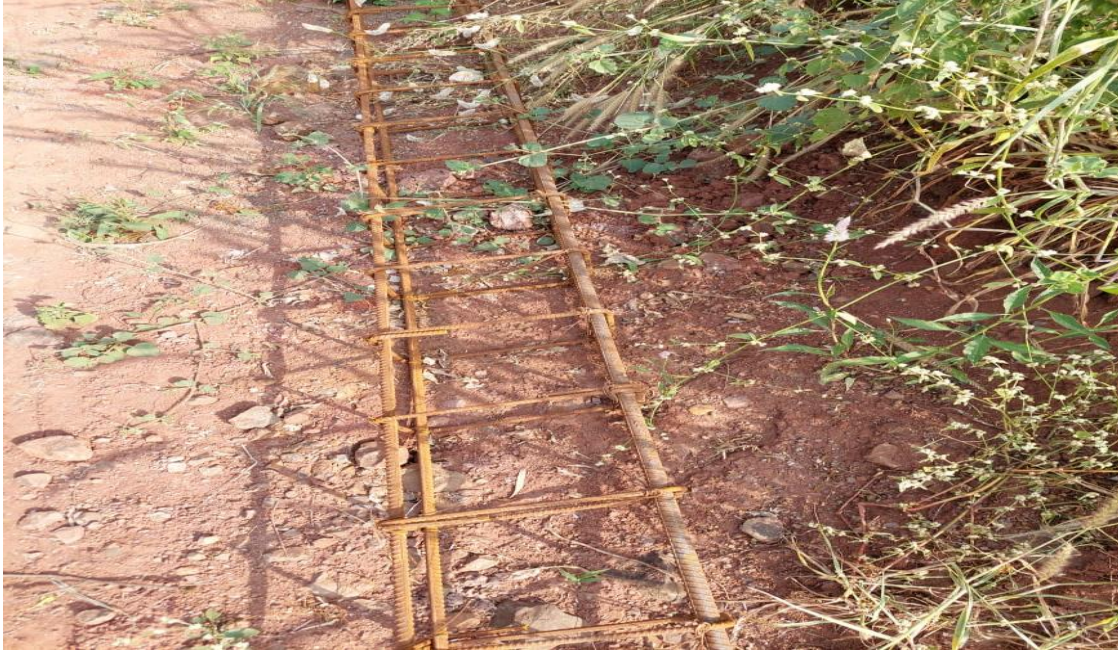
Column reinforcement
