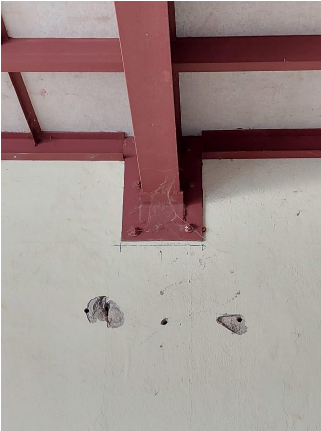
Steel connections with Gusset plate (Bolted connection)
