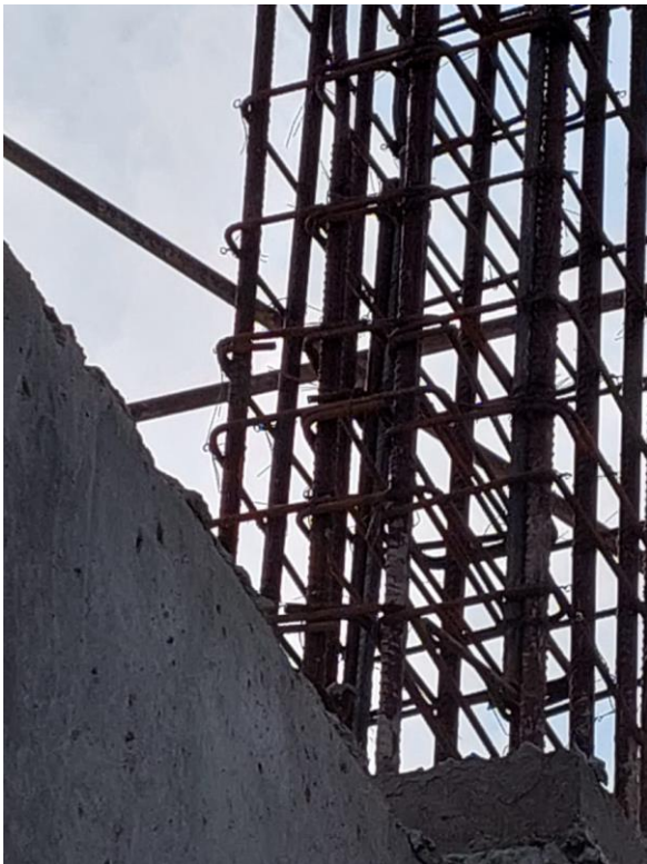
Lap length in column reinforcement
