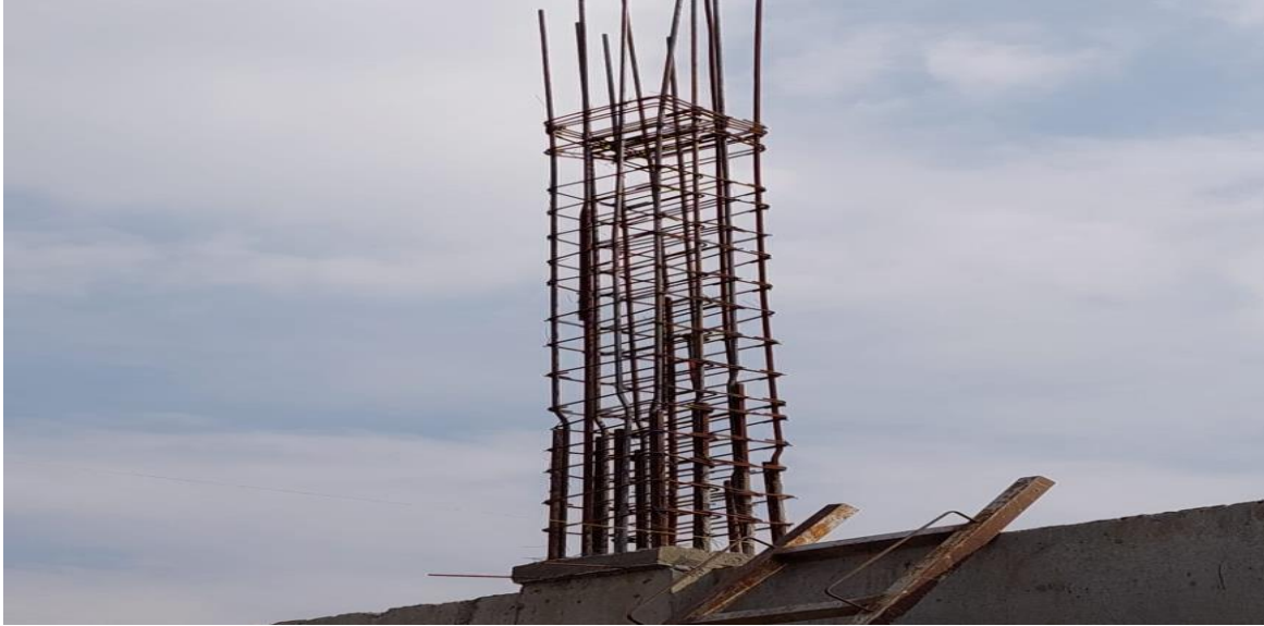
Reinforcement in Column
