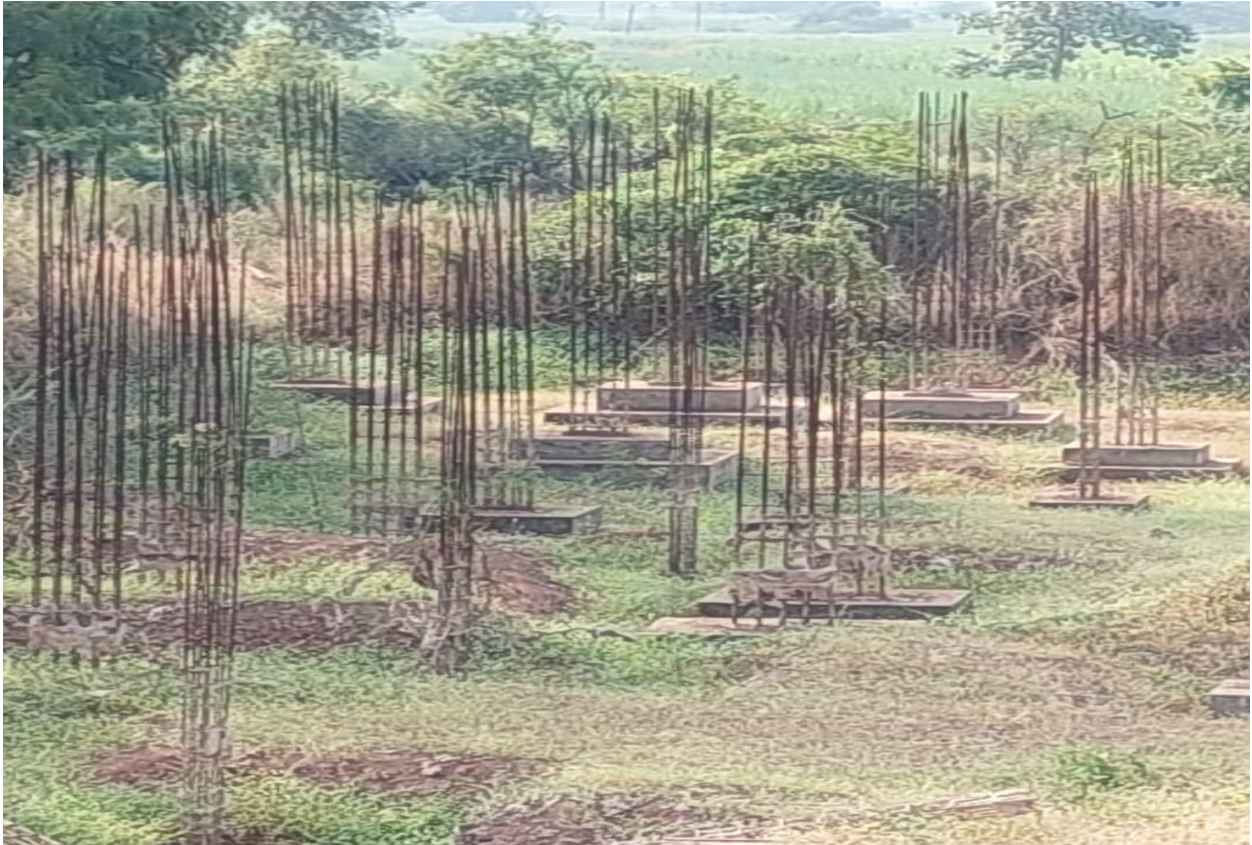
Footing Reinforcement
