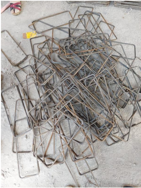
Shear reinforcement ( Stirrups )
