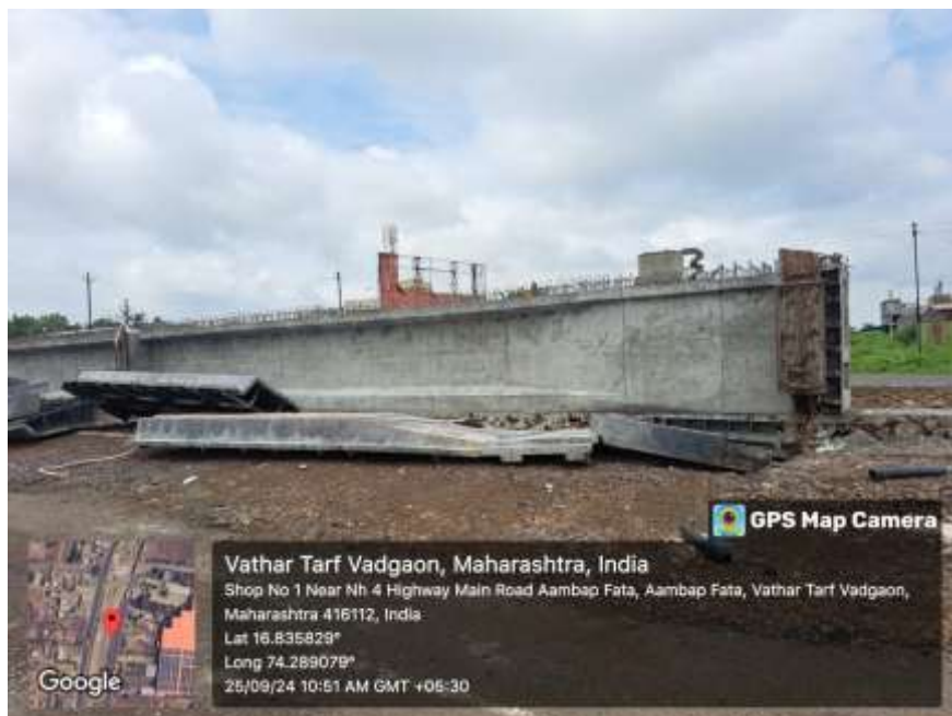
Prestressed RCC blocks used in Flyover
