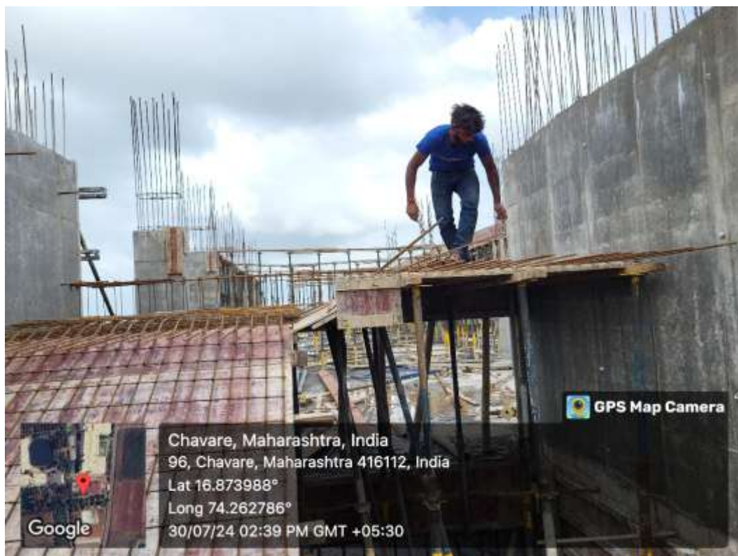
Formwork for Staircase
