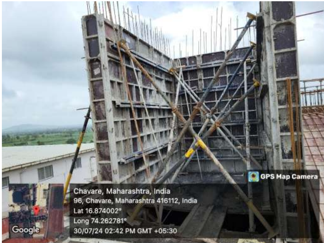
Shear Wall Construction
