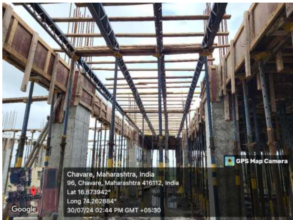
Formwork provided for slab and beam construction
