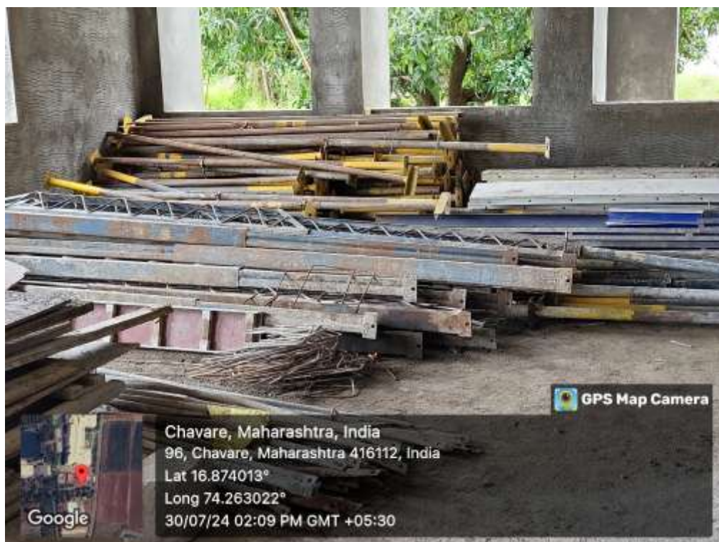
Formwork Channels
