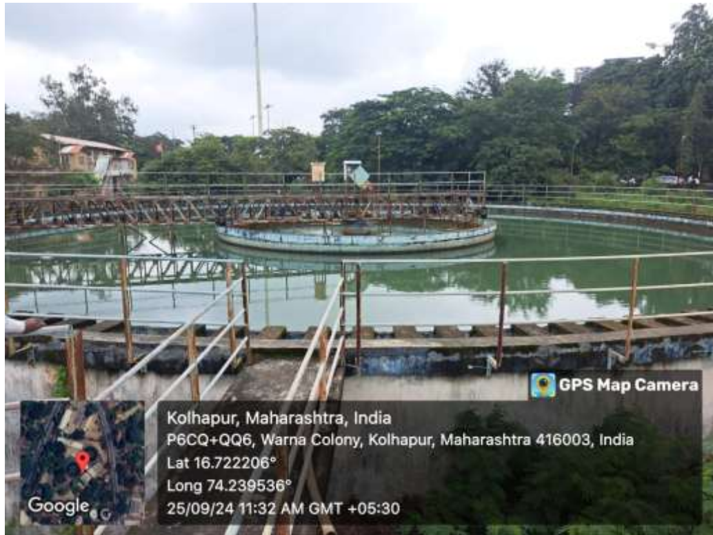
Sedimentation Tank
